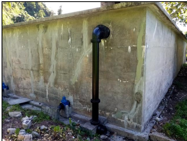
'crackbond' epoxy applied to the 'chip-groved' cracks.
