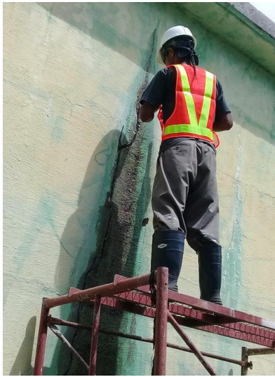
Cracks in raw water tank being prepared for application of 'crackbond' epoxy.
