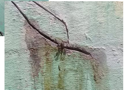
Cracks in raw water tank being prepared for application of 'crackbond' epoxy.
