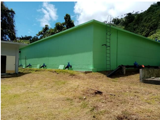
Raw water tank rehabilitated at Pou WTP – July 2020
