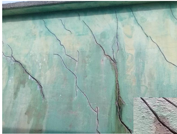
Cracks in raw water tank being prepared for application of 'crackbond' epoxy.
